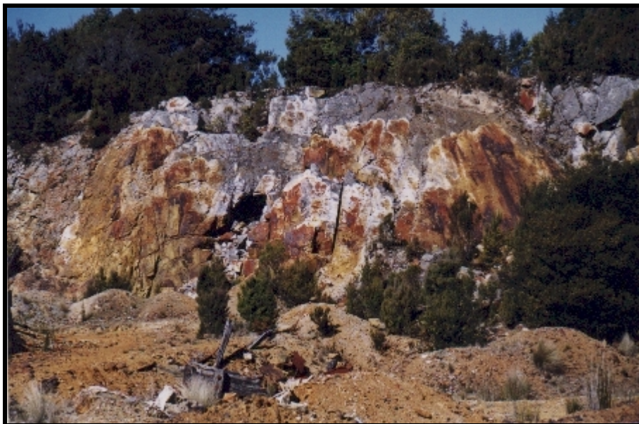
Typical iron oxide coating on a mined rock face resulting from acid generation
